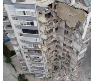
d) Torsional irregularity (Adana)
