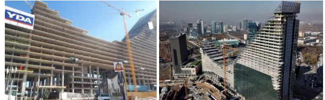
Figure 6: YDA Center under construction [14, 15]
