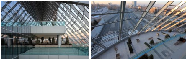
Figure 4: Terraces and façade details [12]
