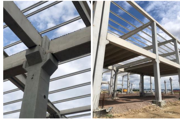
Figure 12: Column-Beam Joints Details
