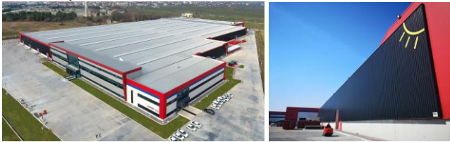
Figure 8: Solar Wall Systems Mounted at Facade, Inan Makina [17]
