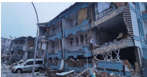
a) Soft storey irregularity-Column rupture (Kahramanmaraş)
