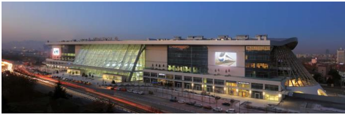
Figure 3: General view of Ankara High Speed Train Station [12]
