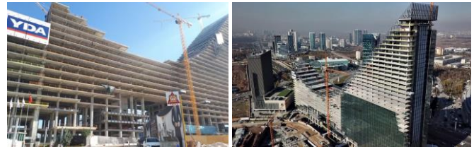
Figure 6: YDA Center under construction [14, 15]
