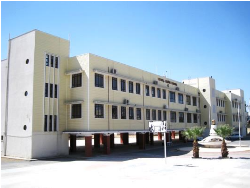
Figure 1. Ataturk elementary school building façade
